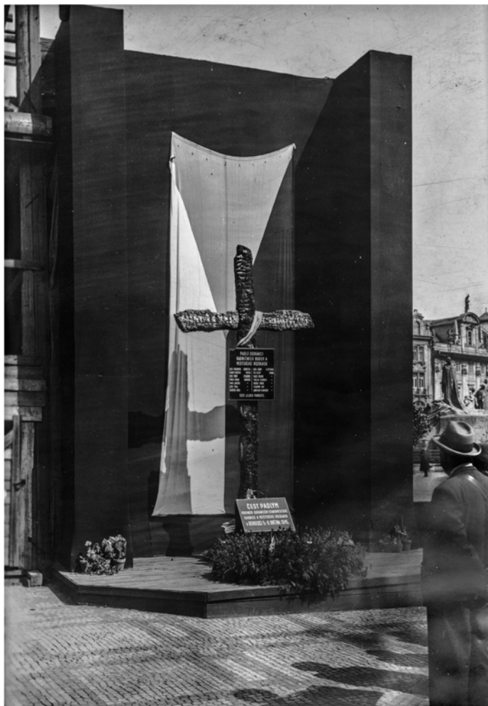
Prague Uprising - May 1945. Makeshift memorial - a cross erected from the beams of the burnt wing of the Old Town Hall with the names of the fallen defenders of the town hall buildings and municipal radio. Taken by Josef Foustecký.
