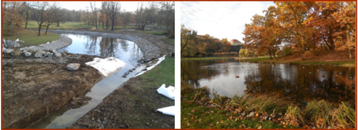
Fig. 13: Enlargement of water bodies at the Stromovka Royal Game Preserve (Project by FLORART, technological design of water bodies by Mr. Jílek)
