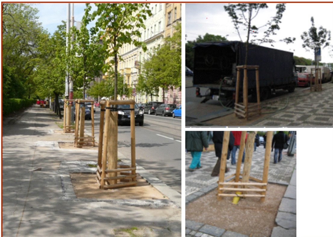
Fig. 8: Total restoration of an alley along the Leger Str. – Jan Želivský St. stretch in Vinohrady Street (Source: Department of Environmental Protection, Capital City of Prague Municipal Office 2007/2008).
