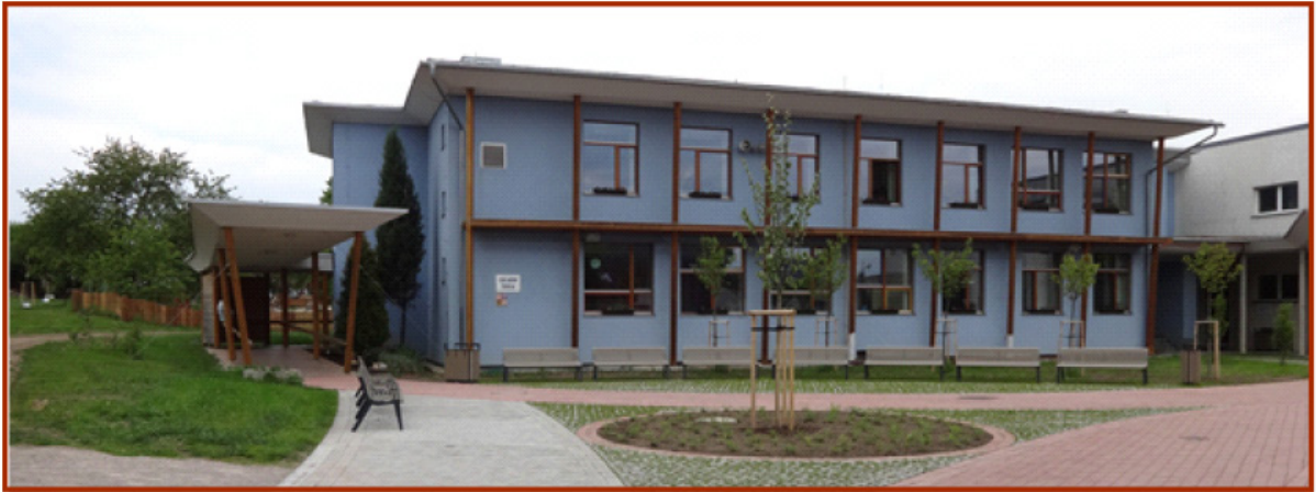
Fig. 29: Passive and low-powered Primary School and Kindergarten with an extensive green roof and a semi-permeable paving in Prague – Slivenec (Source: http://www.skolaslivenec.cz/. )
