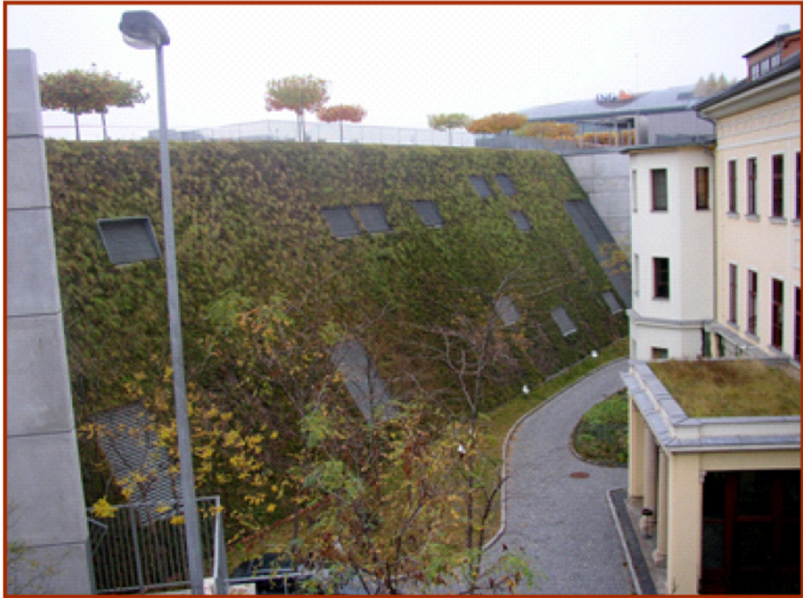
Fig. 31: A vertical green wall at the Smíchov Shopping Centre (© Smíchov Shopping Centre)
